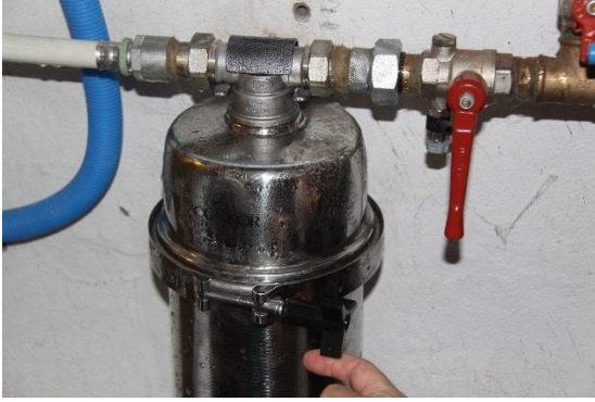
Closed valve (perpendicular to the pipe)
