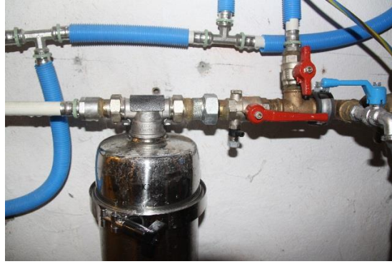
Open valve (parallel to the pipe)
