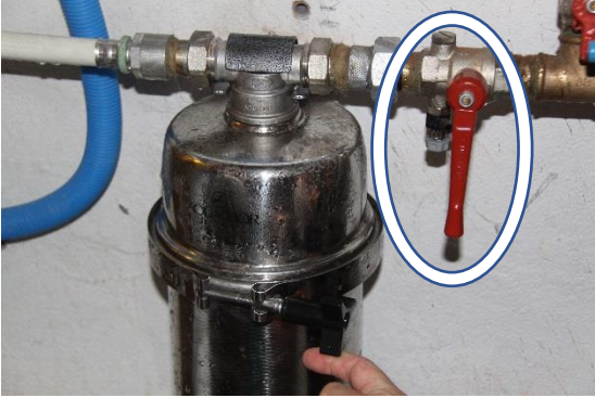
Closed valve (perpendicular to the pipe)
