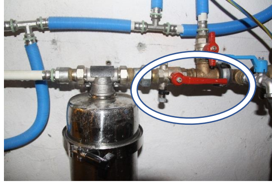
Open valve (parallel to the pipe)
