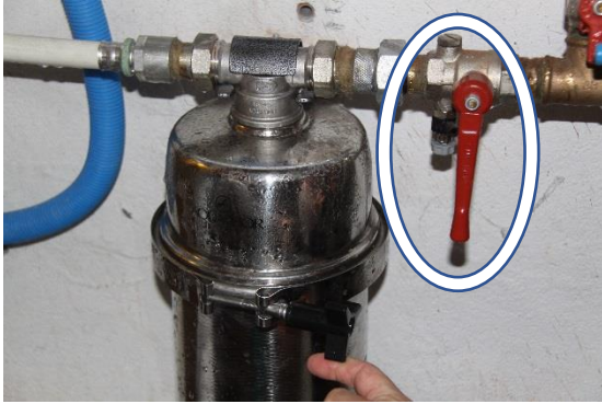
Closed valve (perpendicular to the pipe)
